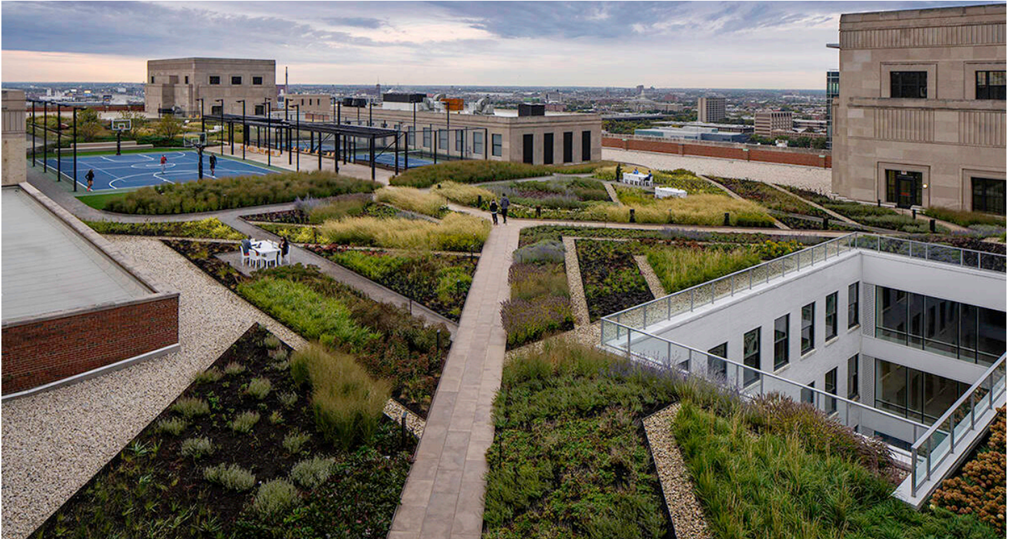
A new living roof designed by Columbia Green Technologies opened on top of the Old Post Office in Chicago. The 3.5-acre rooftop features recreation areas, an amphitheater and running and walking trails. (Tom Rossiter Photography)
