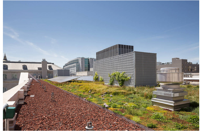
The General Services Administration building at 50 United Nations Plaza features a 14,000-square-foot green roof that reduces the building's stormwater runoff by 75 percent, according to the agency. (Photo by Blake Marvin)
